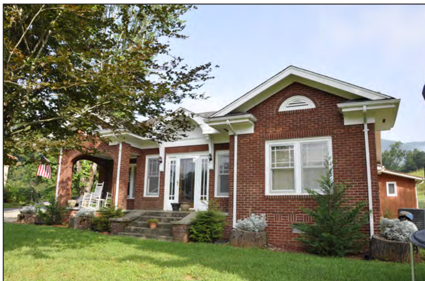
Photograph 2: View of the Jeter Snyder House I; looking north-northwest. (2018)
