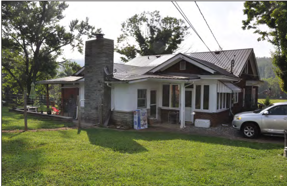
Photograph 3: View of the rear (north) elevation of the Jeter Snyder House I; looking southeast. (2018)
