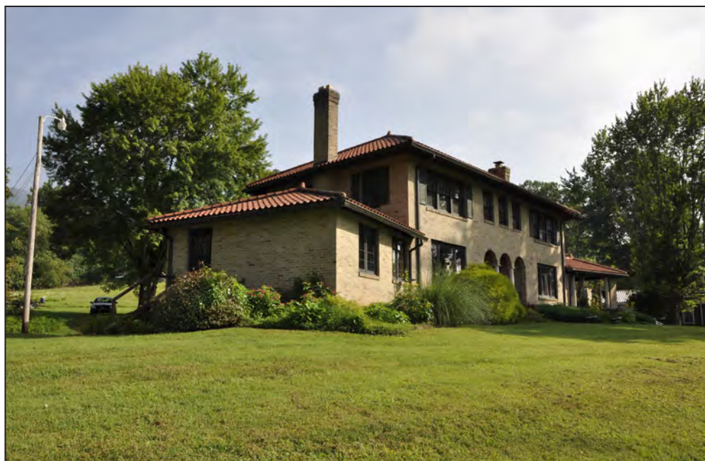
Photograph 16: Oblique view of Jeter Snyder House II looking northeast. (2018)
