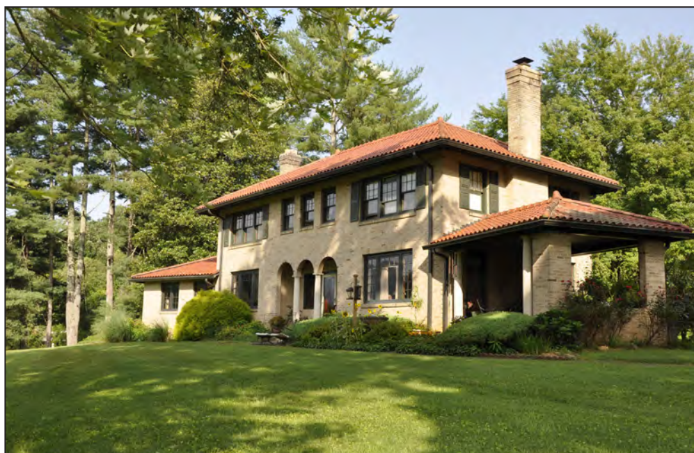
Photograph 15: Oblique view of Jeter Snyder House II ; looking northwest. (2018)
