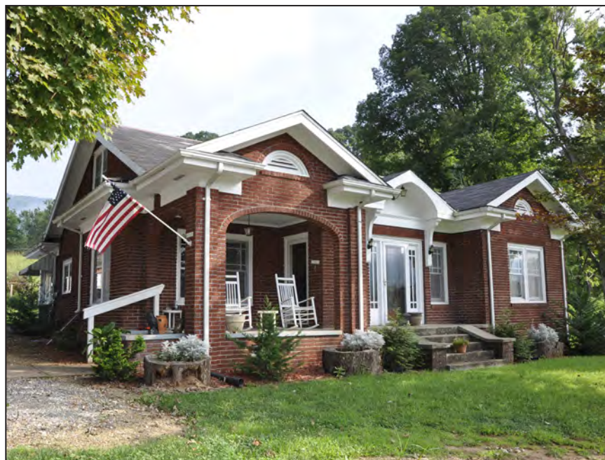
Photograph 1: View the Jeter Snyder House I; looking northeast. (2018)
